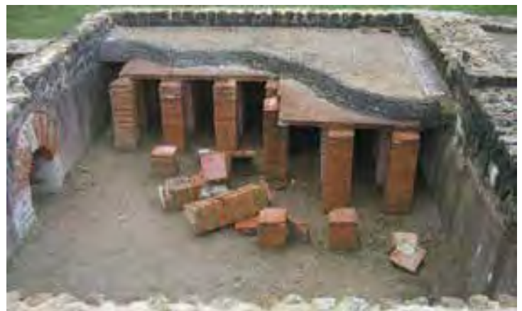
Hypocaust under the floor in a Roman villa in Vieux-la-Romaine, near Caen, France.
