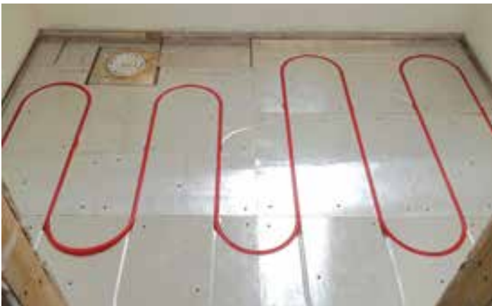
Infloorboard III installed in a bathroom as part of a whole-house application.
